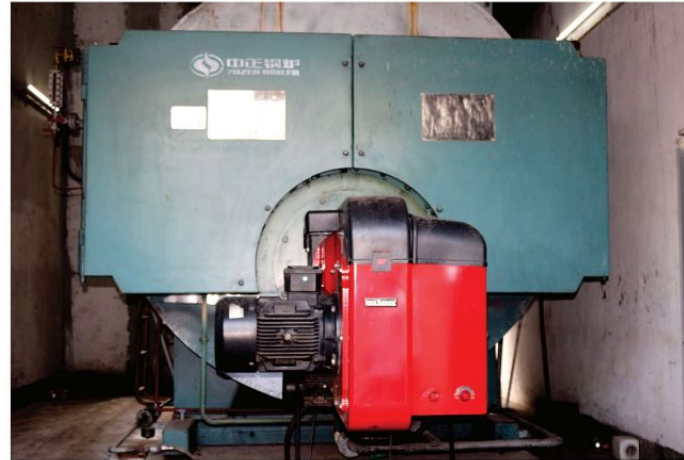
Diesel Boiler
